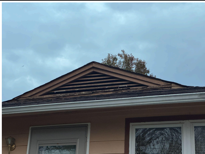
GABLE VENTS & RAKE TRIM (FRONT & REAR) LBP +
