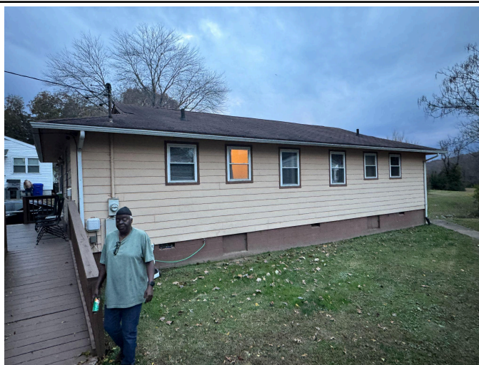
SIDE D EXTERIOR (CRAWL DOOR FRAMES)
